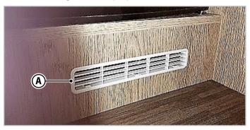
Fig.6.1 - Permanent ventilation openings
